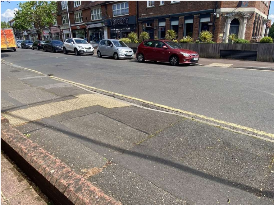
View looking north-east across Green Street from Cheriton Court, showing existing pedestrian dropped kerbs
